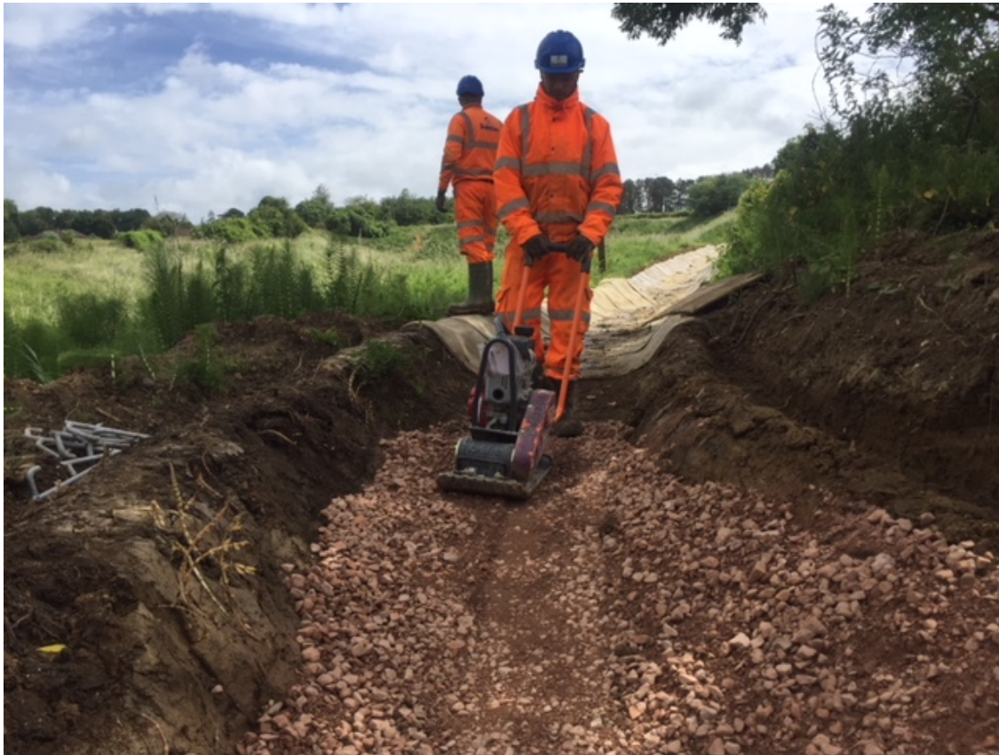
Figure 3: Ditch lining in progress
