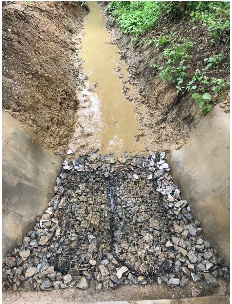
Figure 1: Rock rolls as scour protection to outlet headwalls
