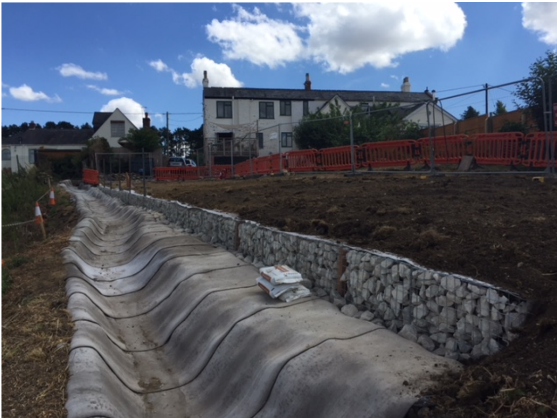
Figure 4: Completed top of cutting ditch
