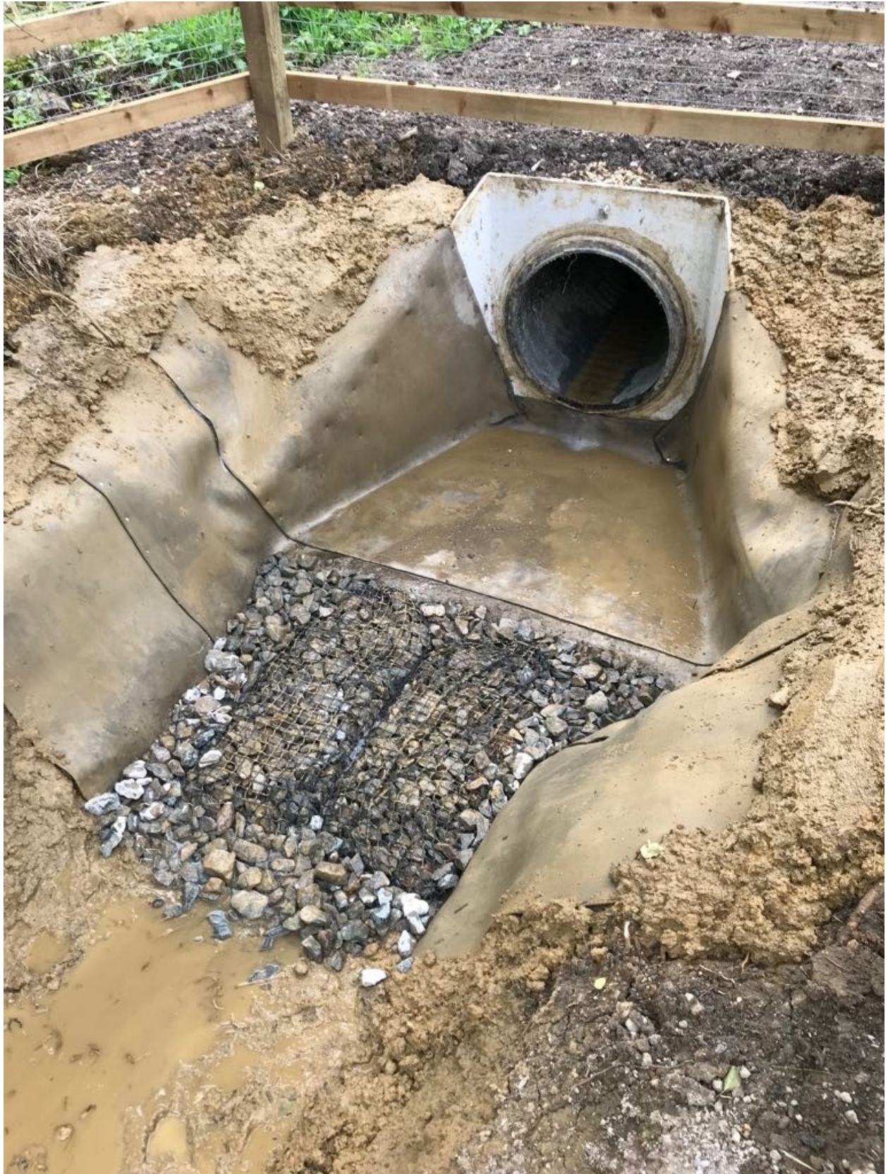
Figure 2: Outlet featuring concrete canvas and rock rolls
