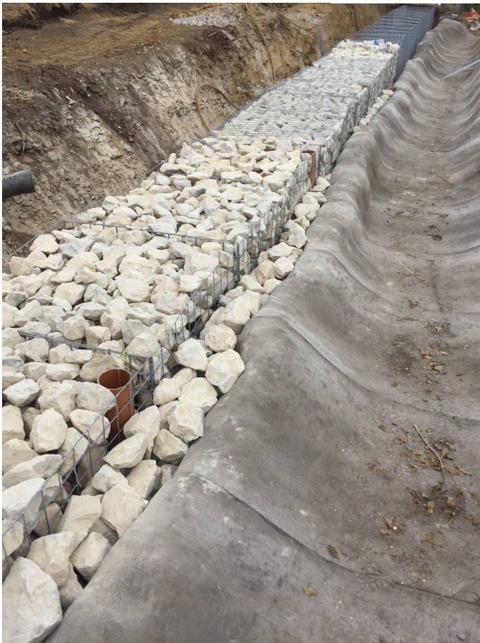
Figure 6: Gabions to enhance ditch construction
